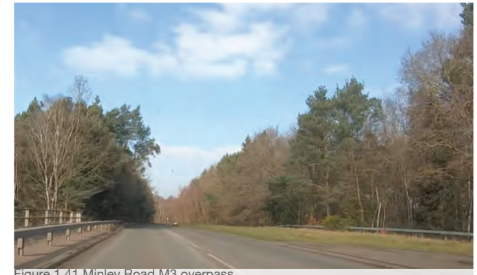
Figure 1.41 Minley Road M3 overpass
