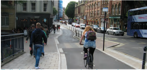
Fully kerbed segregated cycle track
